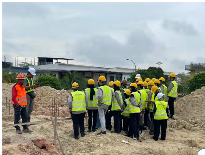
Fig. 3 Students observing the Excavation work.
